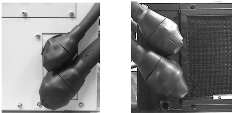
**Figure 3-25 Keeping Copper Piping and Quick Thread Connector Insulated**
