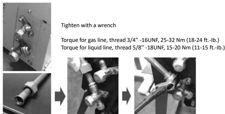
**Figure 3-26 Tightening the Connectors of The Condensing Unit**
